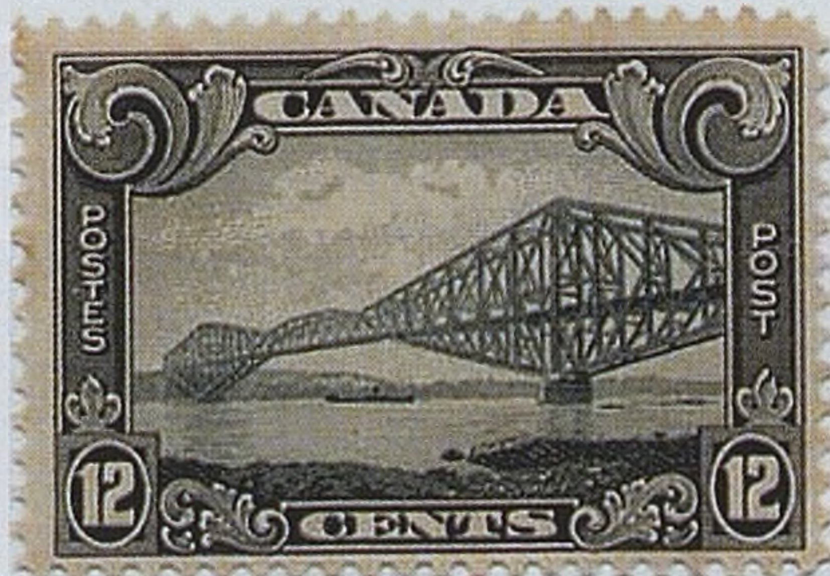
■ The Quebec City Bridge, 1917
